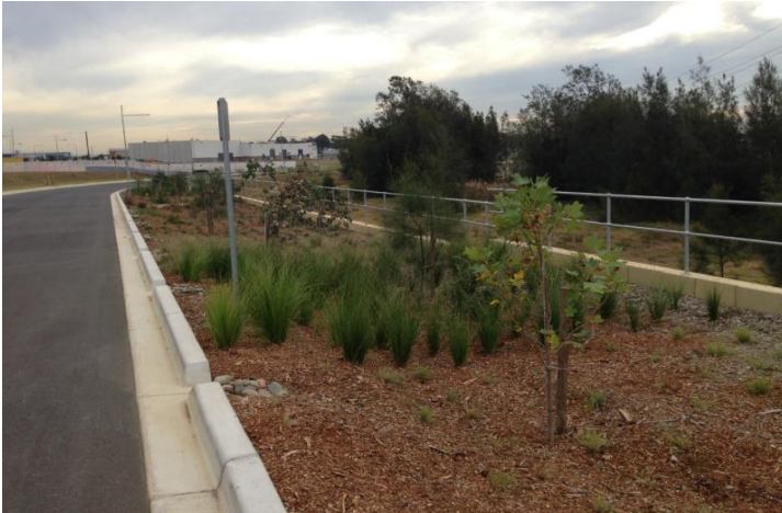
Figure 6: Bioretention System
